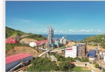
Great Lakes Plant Annual Capacity (mt): 1.5 Commissioned: December 2022
