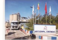
National Cement Plant Annual Capacity (mt): 1.3 Commissioned: November 2022
